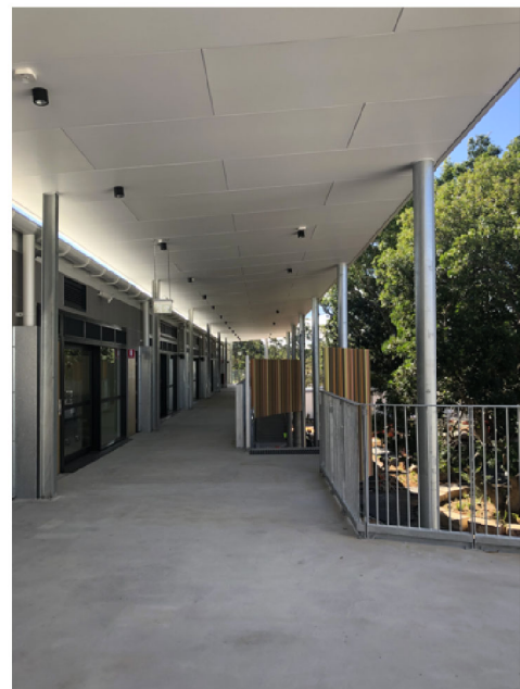
FC SOFFIT - MAIN ROOF WALKWAYS PAINTED DULUX 'CEILING WHITE'
