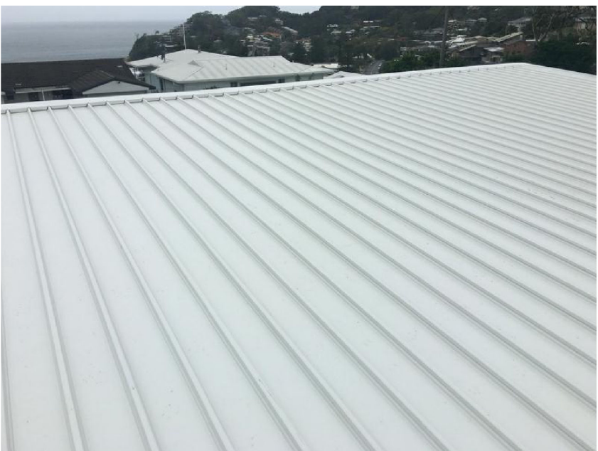
LYSAGHT KLIPLOK ROOFING, COLORBOND SURFMIST
