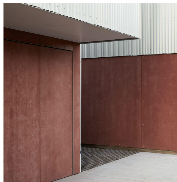
'RUST' CFC CLADDING
