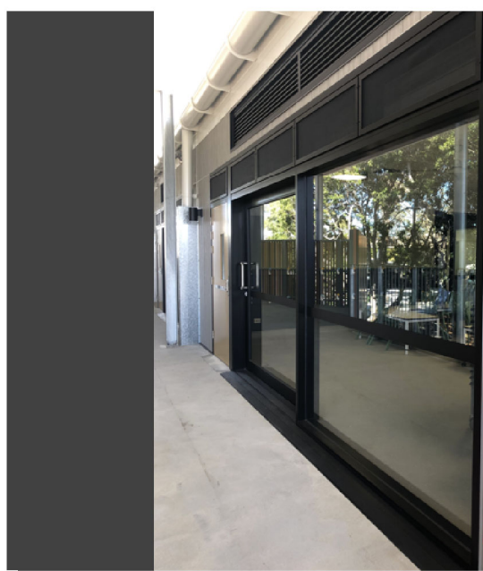
POWDERCOATED ALUMINIUM WINDOW FRAMES, BLACK (MONUMENT)
